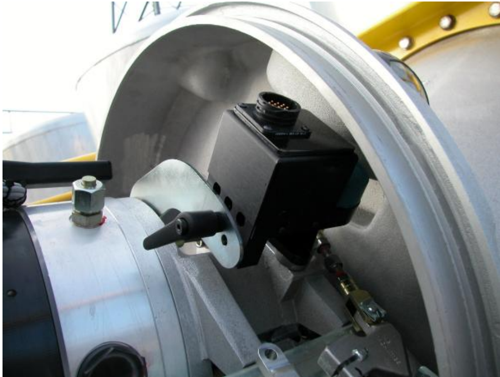
Rotary Transducer on ABB HMB Mechanism
