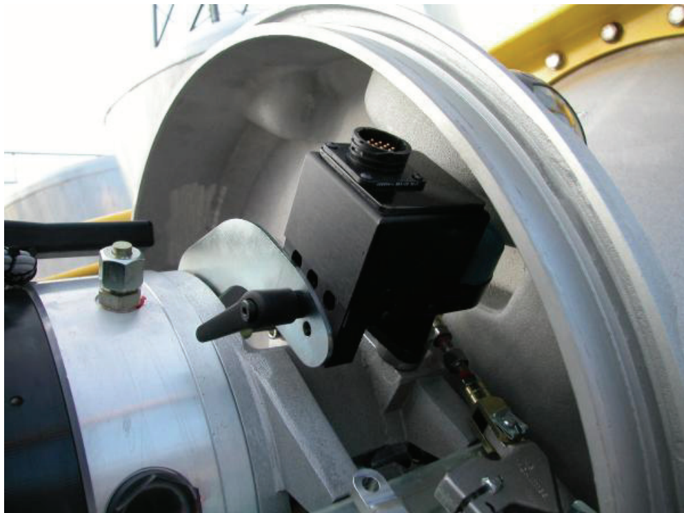
Rotary Transducer on ABB HMB Mechanism
