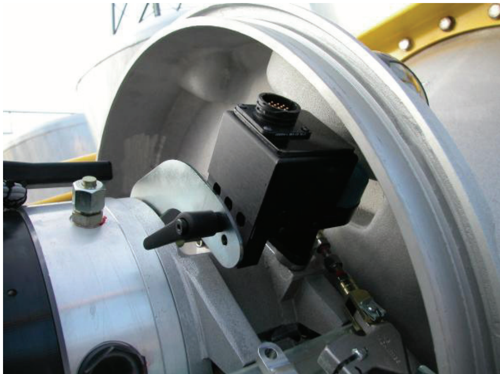
Rotary Transducer on ABB HMB Mechanism
