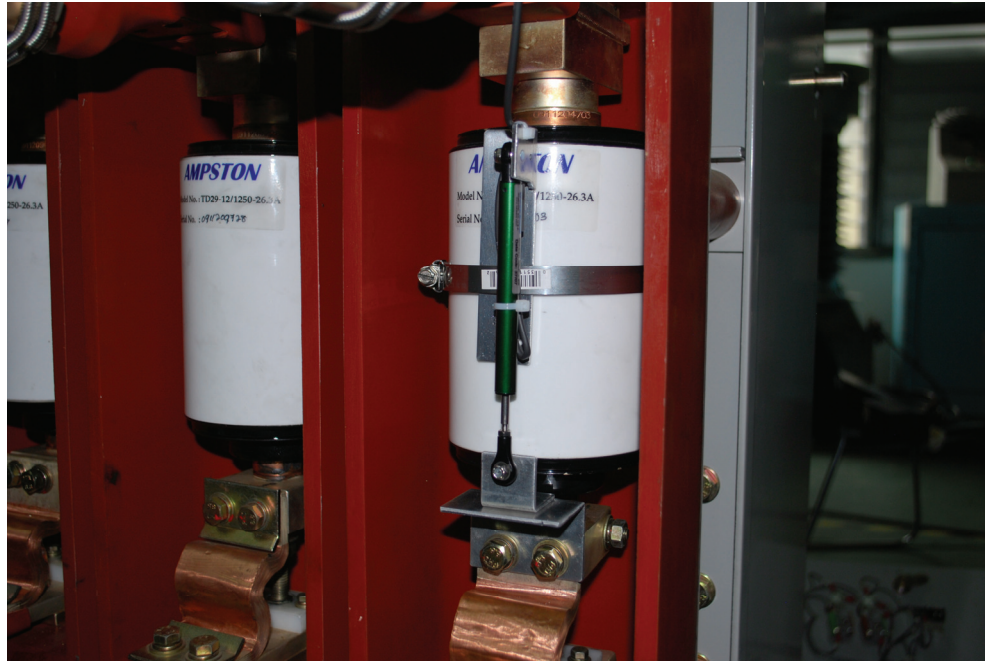
Resistor Transducer on Vacuum Circuit Breaker
