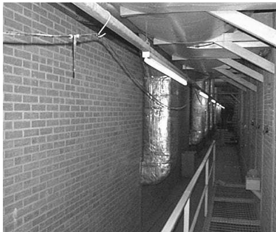
Low-loss modular-array antenna installed along a kiln.
