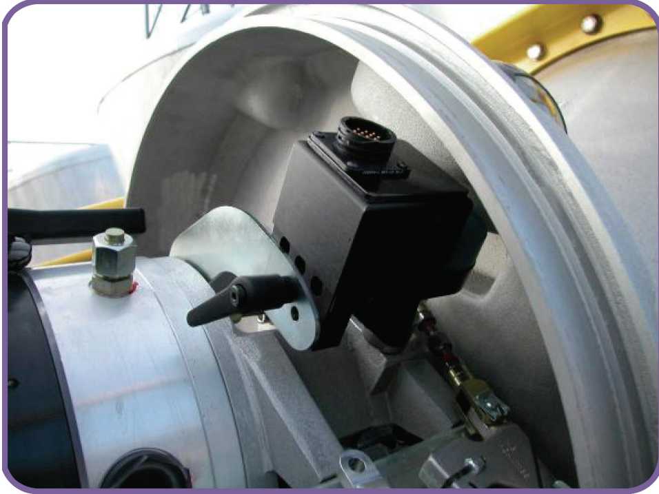
Figure 28. Rotary Transducer on ABB HMB Mech
