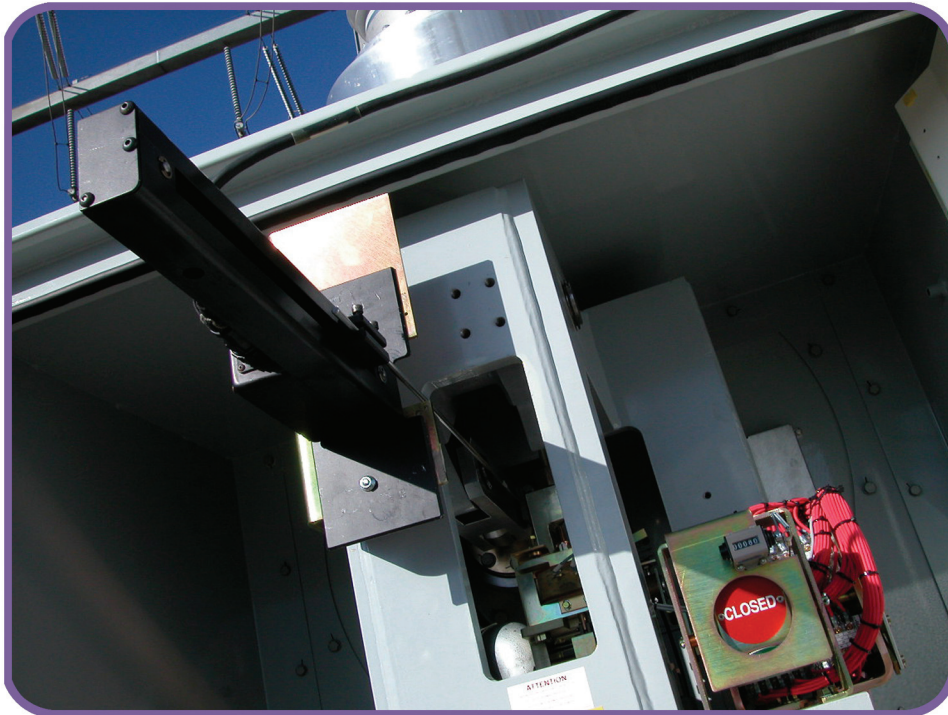
Figure 33. Linear Transducer on Mitsubishi 500-SFMT
