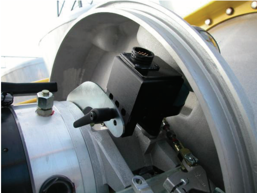
Rotary Transducer on ABB HMB Mechanism
