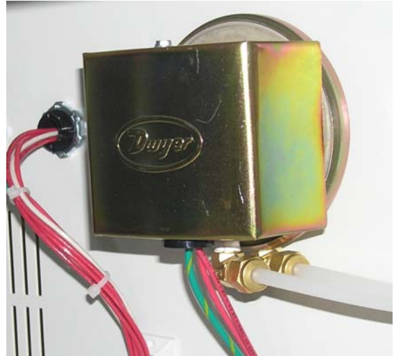
DIFFERENTIAL AIR PRESSURE SWITCH
