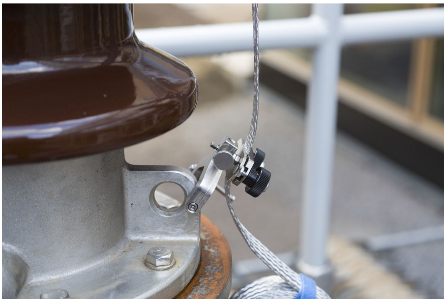
Figure 5-6: Alternative way of fastening the screw clamp
