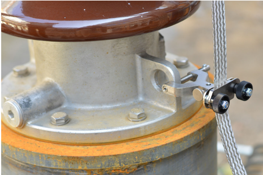
Figure 5-5: Fastening the screw clamp
