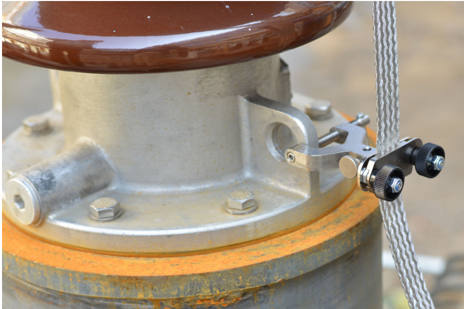
Figure 4-5: Fastening the screw clamp
