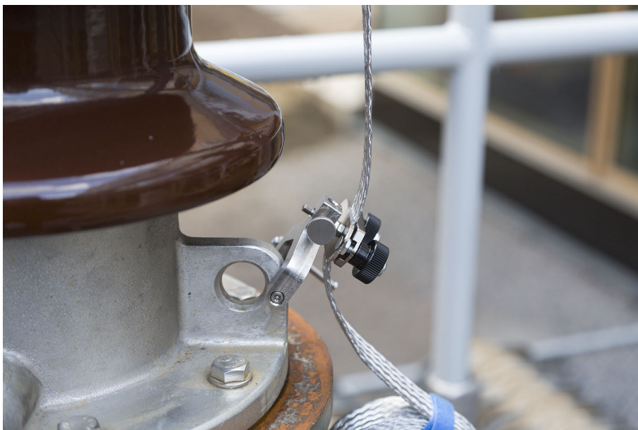
Figure 4-6: Alternative way of fastening the screw clamp
