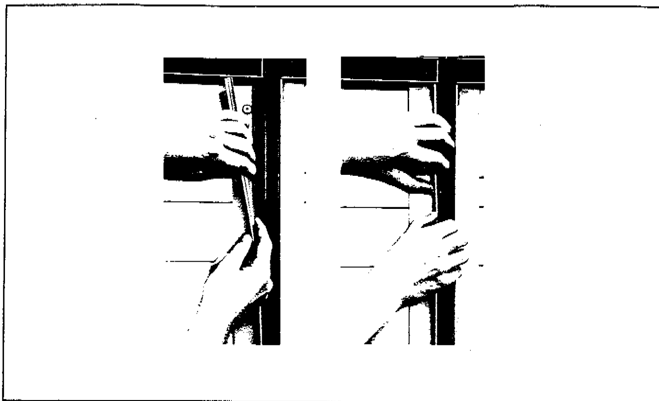
Figure 4-5. Plastic Trim Strip Installation
