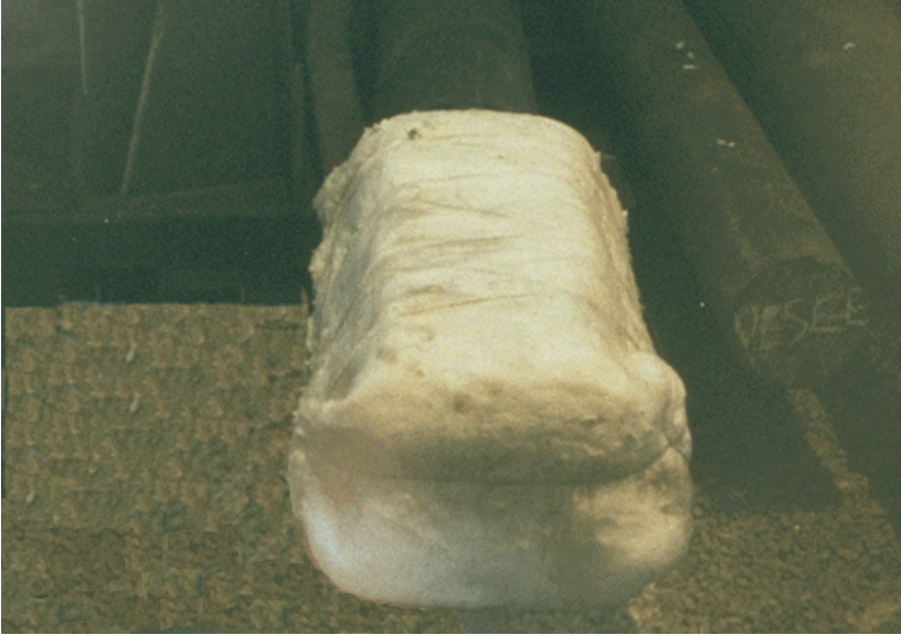
Photograph 25 The final insulation layer is secured with nickel wire
